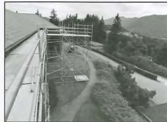
Reroofing the southern end of the minor seminary
