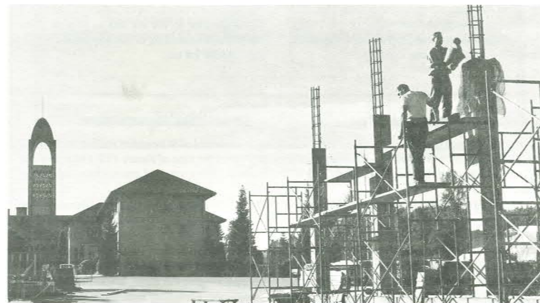
Building the Gymnasium
